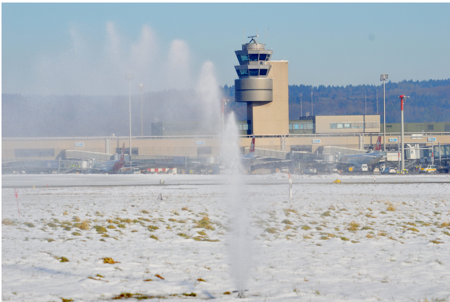
The sprinkler system sprays de-icer runoff onto grassed areas.
