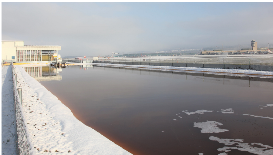
Highly concentrated de-icer runoff is collected in a basin then distilled in the airport's own plant.
