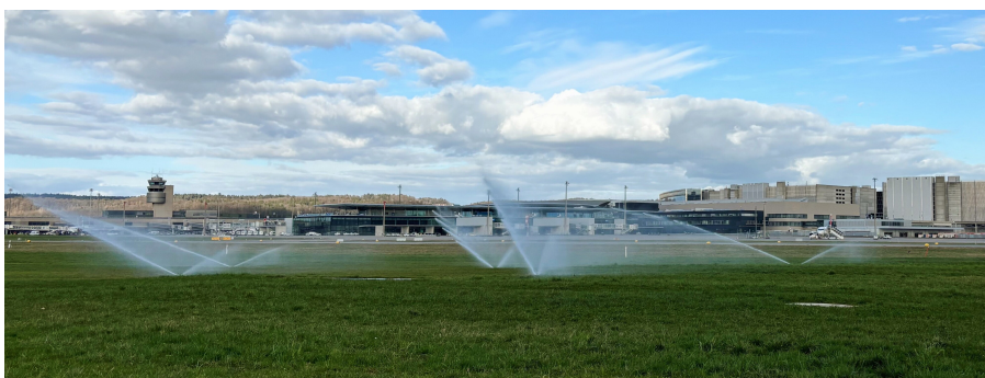
The sprinkler system sprays wastewater containing de-icing agents onto green spaces. The water is cleaned as it percolates down through the soil.
